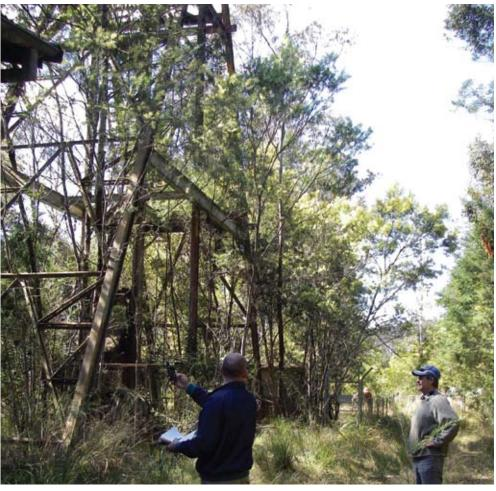
An historic head frame at Bielsdown, which was used for a shaft that was previously sunk to a depth of 165 metres.
